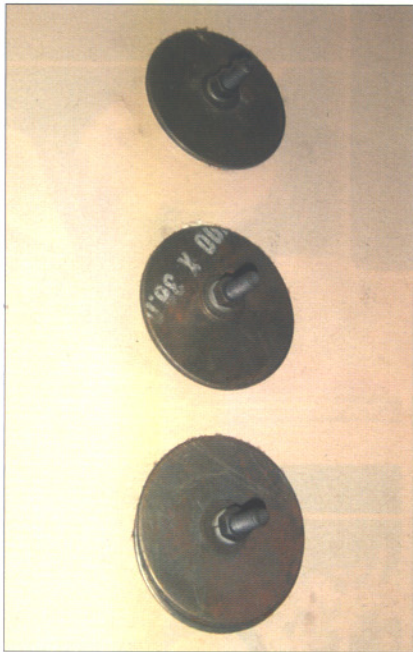
Five-inch diameter washers reinforcing three wallmount bolt fasteners installed through the wall.
