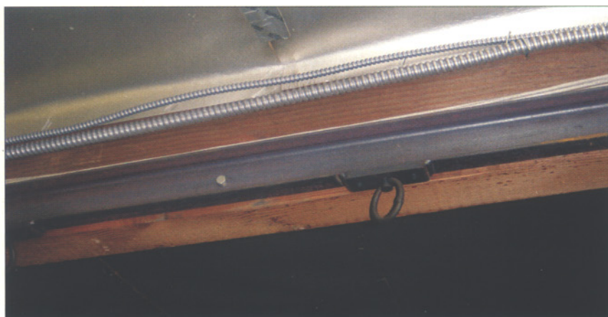
ASTM C3X5 Channel reinforcement attached to a ceiling joist.
